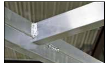
Welded, Integrated Roof Structure
